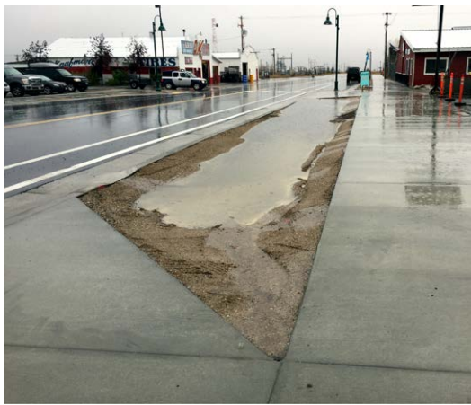
Green stormwater treatment. Upper left, before improvements, rainwater flooded the street and sidewalk; above left, during construction, rainwater pools in bioretention basins. Right, basin landscape plant materials will grow over time, treating runoff. Below, structural Silva cells are placed in tree wells and under the sidewalk, allowing trees to flourish and providing in-ground infiltration of stormwater rather than surface runoff.
