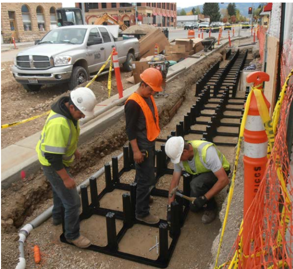
Green stormwater treatment. Upper left, before improvements, rainwater flooded the street and sidewalk; above left, during construction, rainwater pools in bioretention basins. Right, basin landscape plant materials will grow over time, treating runoff. Below, structural Silva cells are placed in tree wells and under the sidewalk, allowing trees to flourish and providing in-ground infiltration of stormwater rather than surface runoff.
