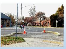
A traffic circle or mini-circle can be used at intersections on low volume, local roads. Without realigning the roadway, adding a small island and vertical element in the center of the intersection (right) causes traffic
