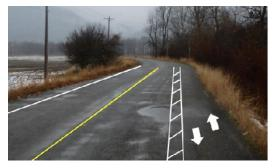
provide physical separation between the travel lane and the marked pedestrian/bicycle lane. Such a path can be five to eight feet wide, with a marked line or buffering stripe (e.g. 12-inch striping).
