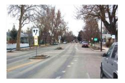
Guidance on traffic lane widths show they can be as narrow as nine feet in appropriate locations.
